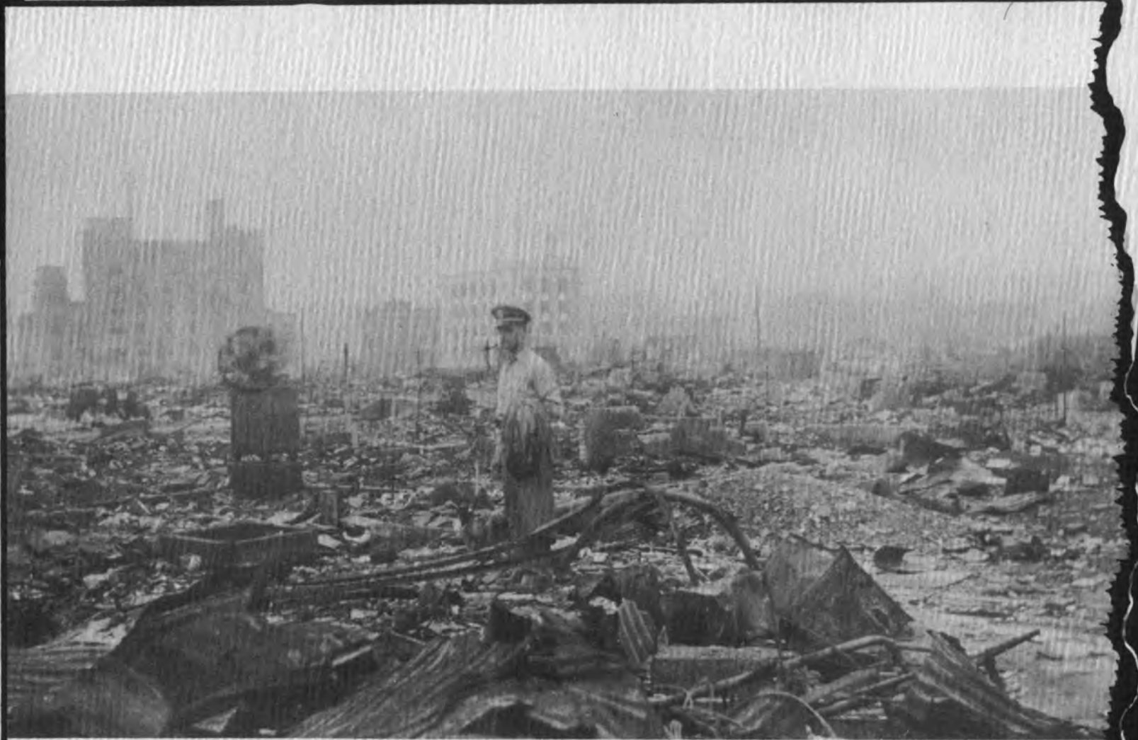
Tokyo and Yokohama
