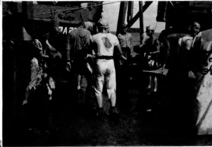
GOING THROUGH THE MILL
